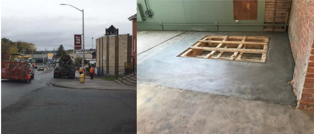
In the gym all the rough-in plumbing work was completed and the excavated areas were back filled and concrete poured to provide a continuous flat floor. The next step will be the floor finishes, which will only occur when the project has progressed to the finishing stage.
