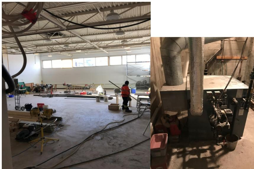
The mezzanine floor has been installed in preparation for the installation of the HVAC equipment. In order to get the equipment into the mezzanine, scaffolding was set up in the alley to allow the Masons to create a wall opening at the mezzanine level mechanical space. Once the masonry work is complete a steel door frame with double doors will be installed to provide mechanical room access for our equipment installation.
